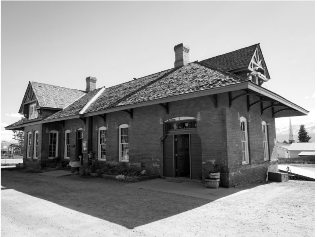
The historic Colorado & Southern passenger depot is still serving its original purpose.
