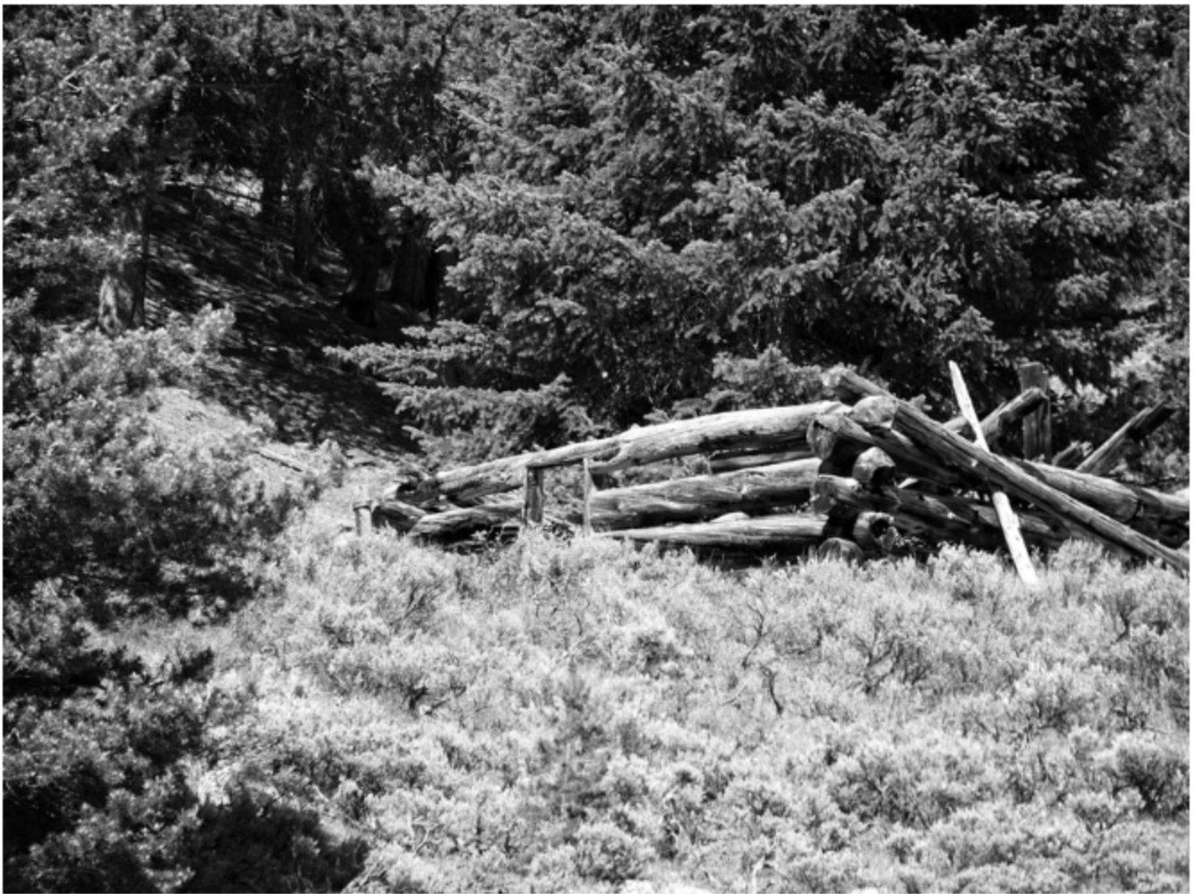
The remains of an old cabin that was built to house track crews.
